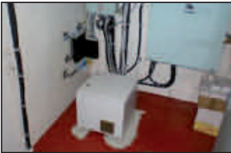
DC-UPS EN60945 marine approved for VDR (black box) systems at large ships.
